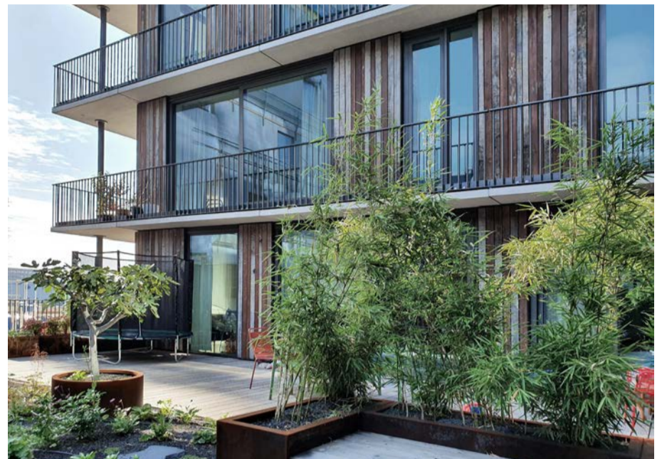
The collective roof garden functioning as a water buffer and adding biodiversity
