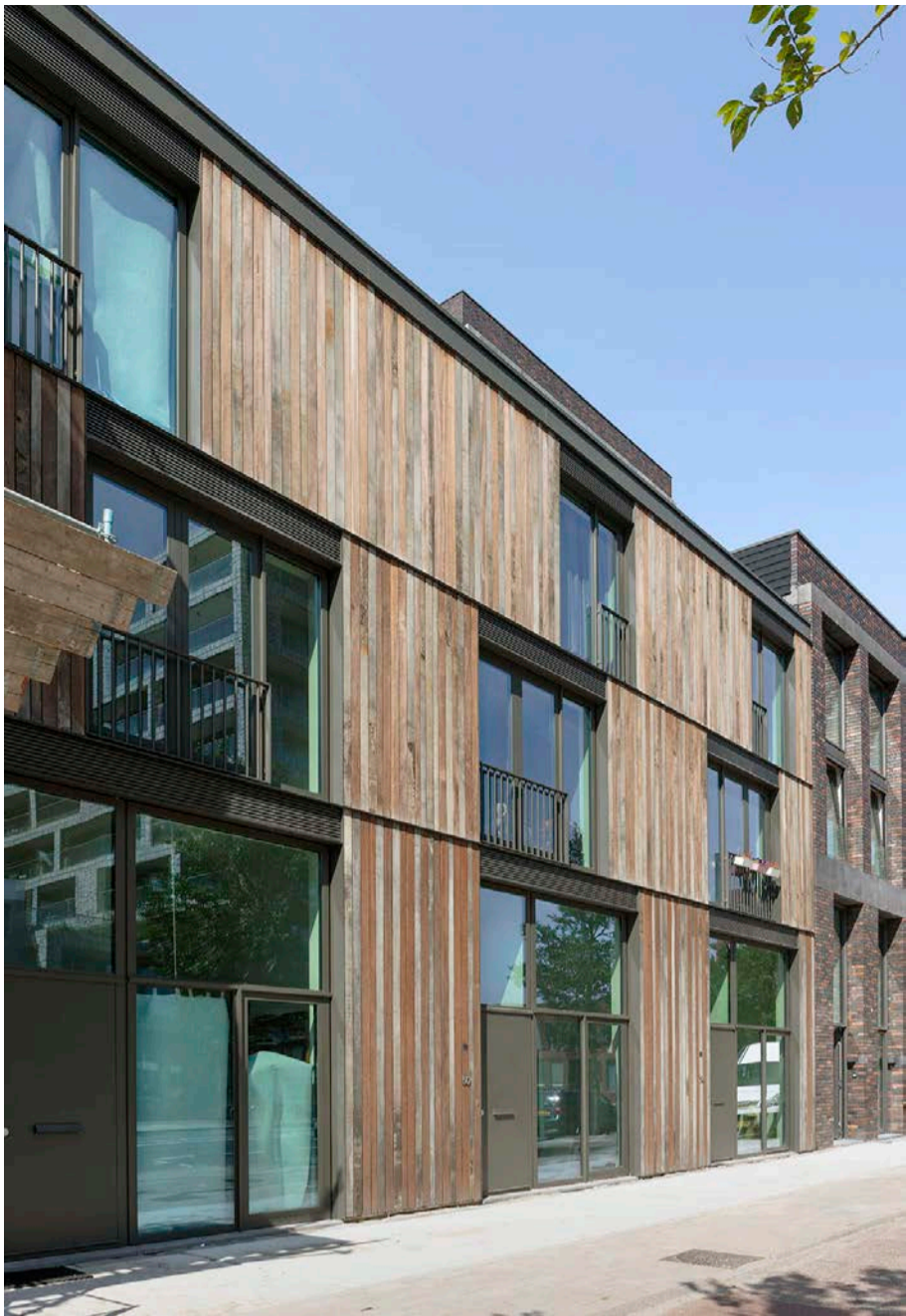
The Azobé wood, formerly used in Dutch quay walls, gets a second life within the facade
