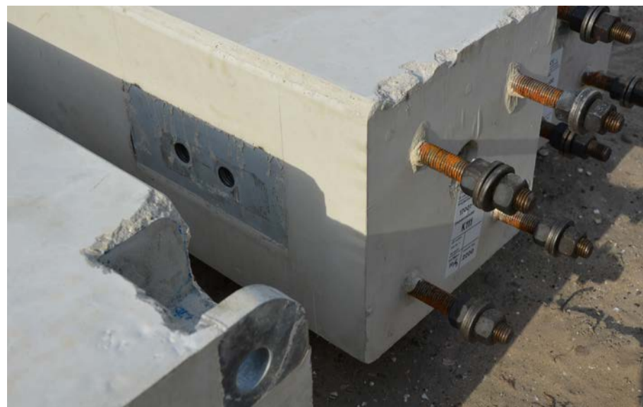
The connection of the demountable concrete columns
