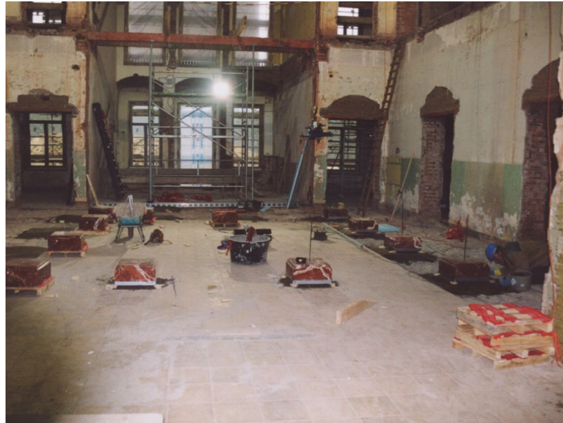
The ground floor at the start of the construction works
