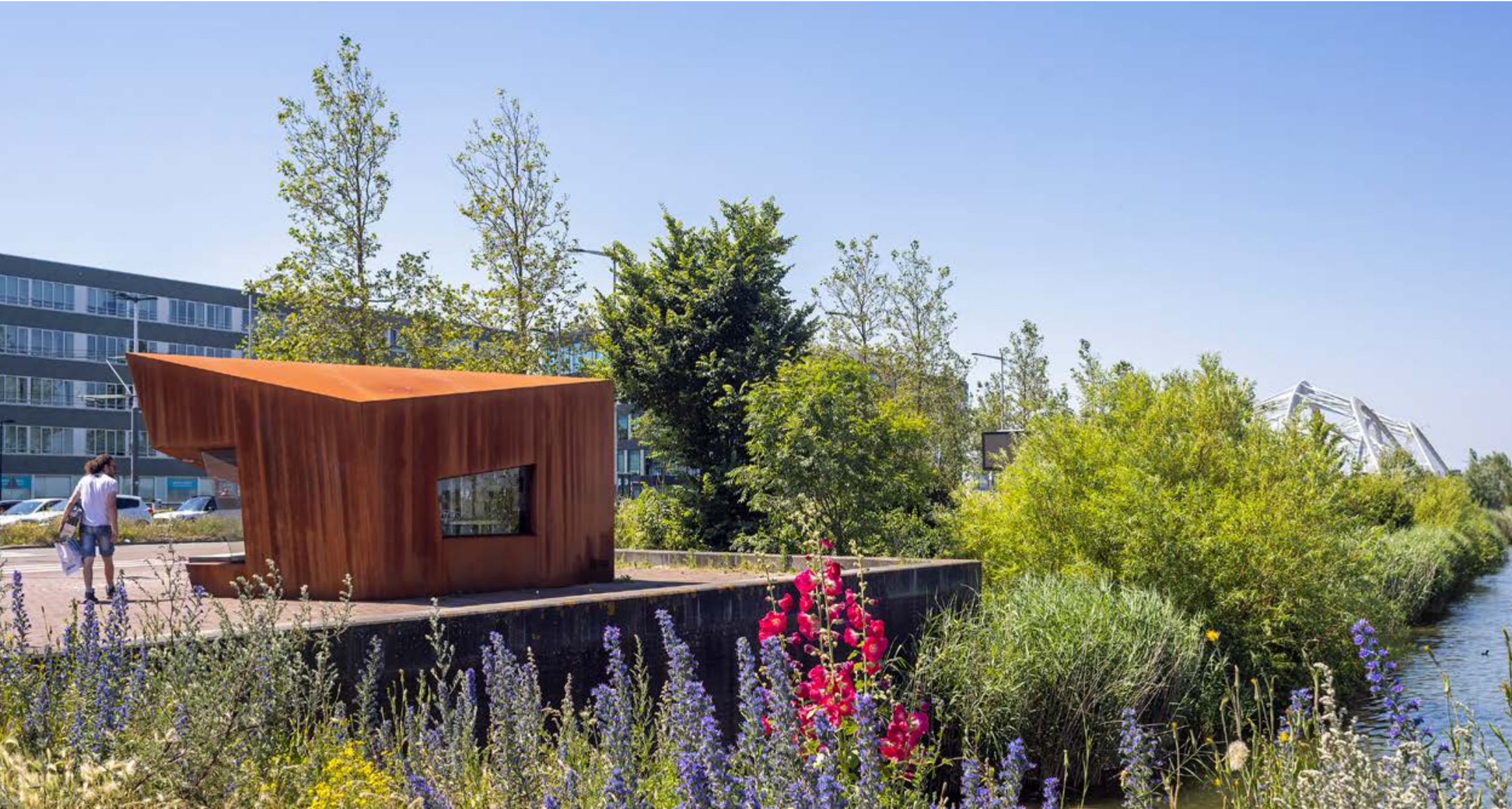
Warmte Overdracht Station - Amsterdam
